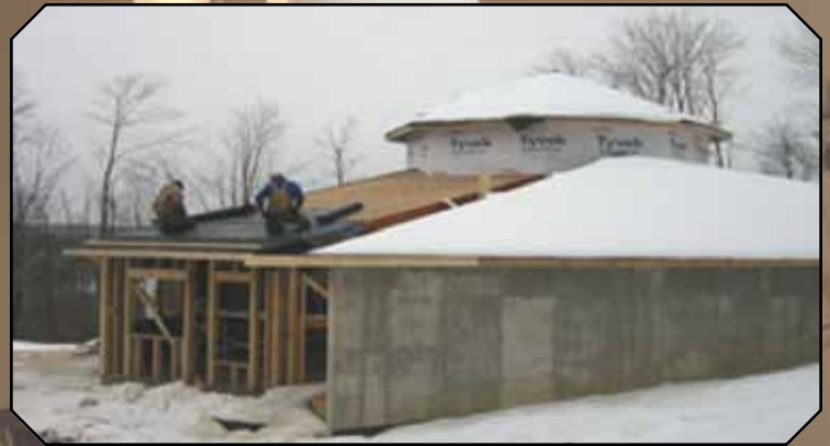
On-Site Built Building Weather
